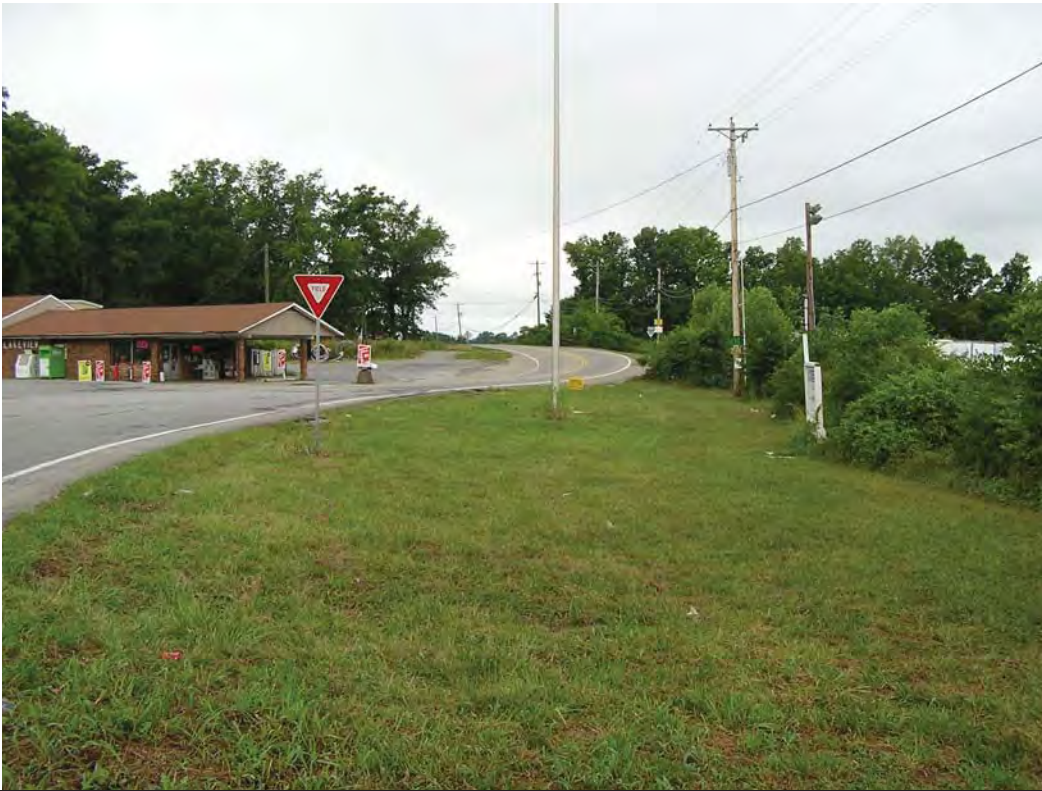
Photo 1: STA 364+50 LT. View of SR-333 (Topside Road) facing west. Photograph taken 7/10/14.
