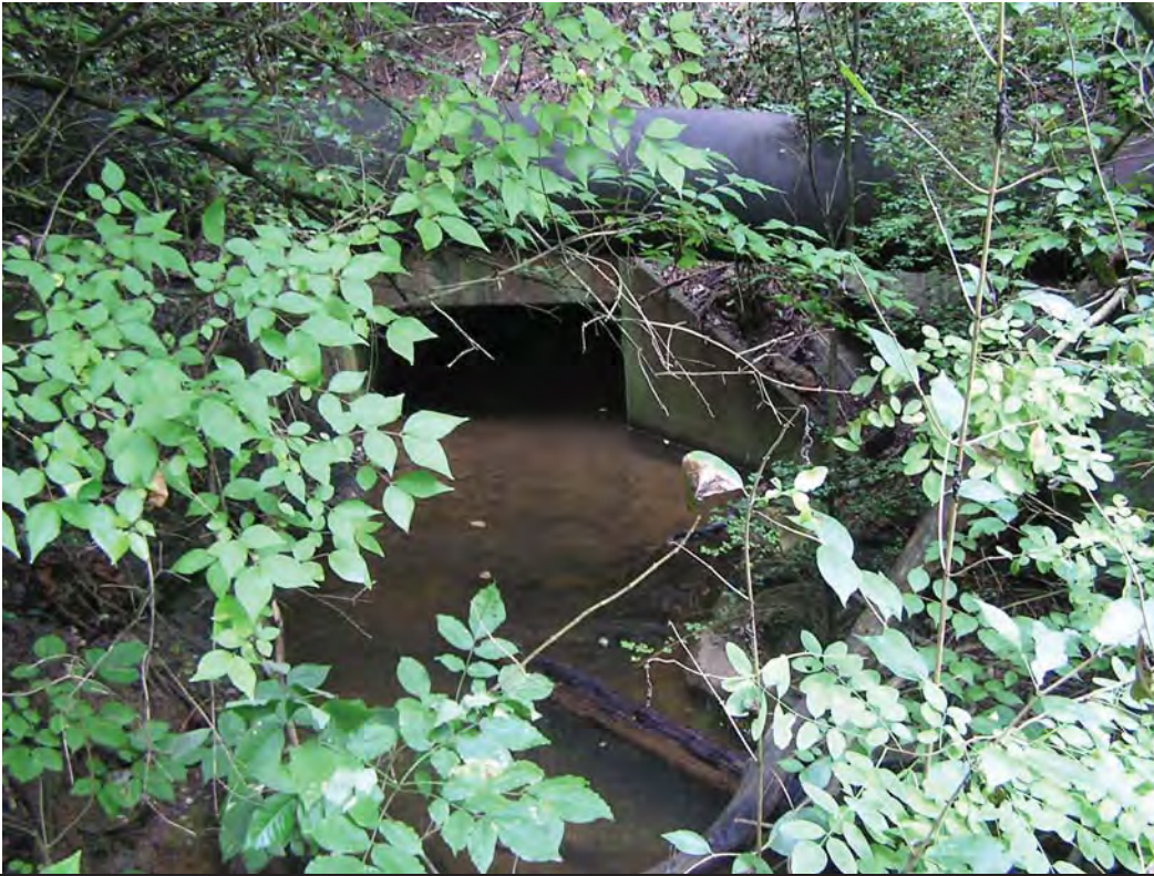
Photo 5: STA 367+25 RT. View of STR-1 facing west (upstream). Photograph taken 7/10/14
