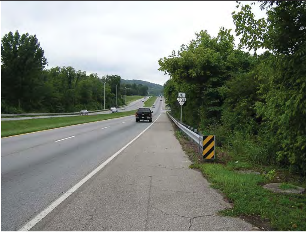
Photo 3: STA 369+00 LT. View of SR-115 (Alcoa Highway) facing south. Photograph taken 7/10/14.
