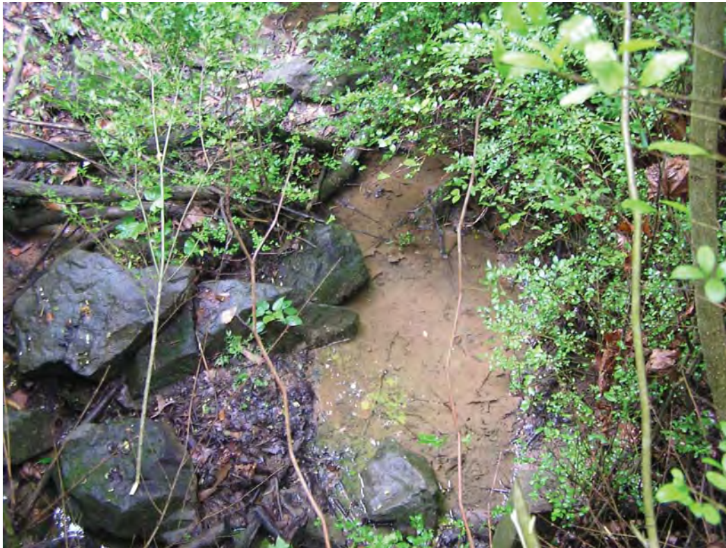
Photo 4: STA 367+25 LT. View of STR-1 facing west (upstream). Photograph taken 7/10/14.
